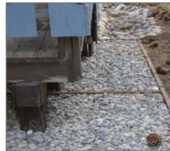
Gravel area under a gutterless roof
