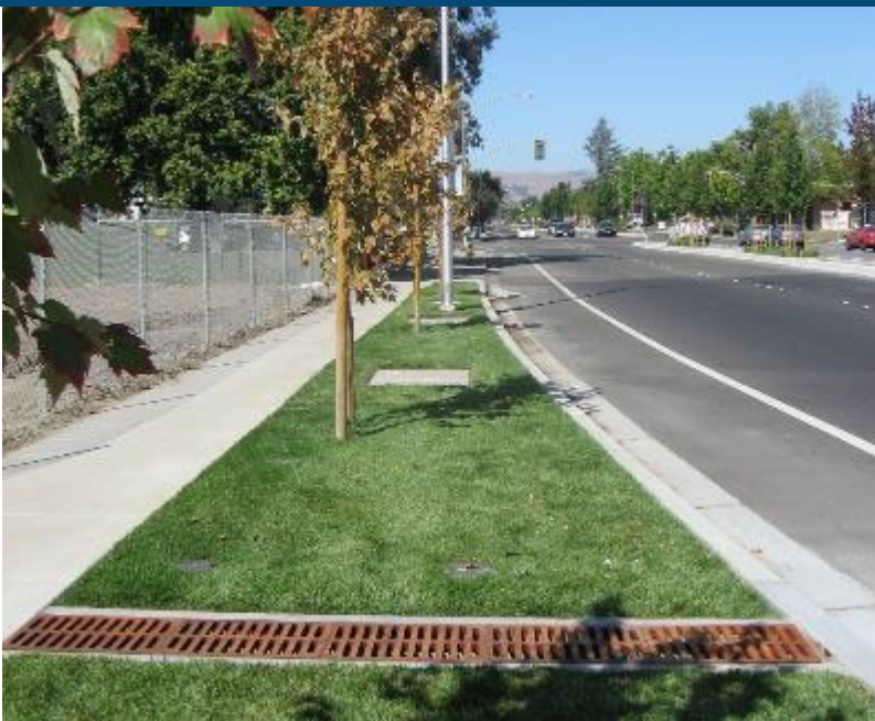
Figure 8-16. Non-proprietary tree well filters in Fremont
