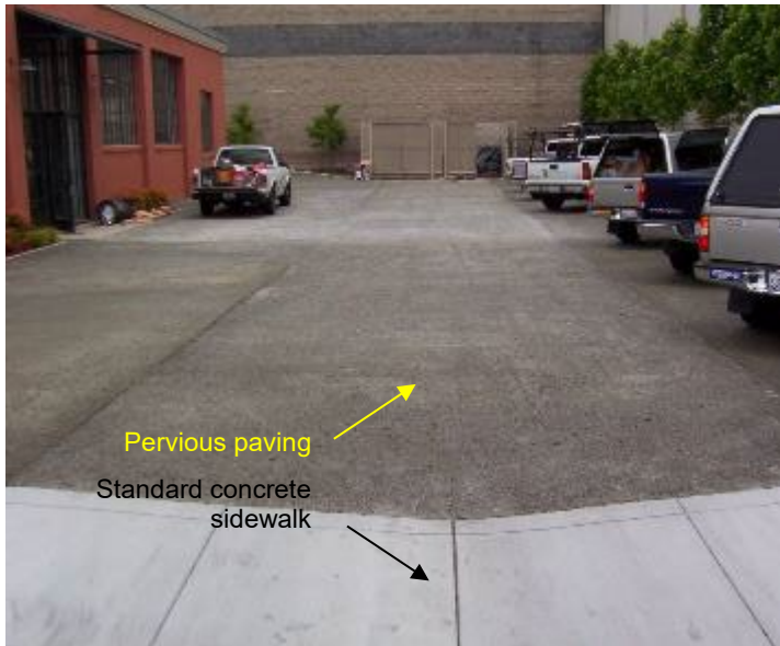
Figure 8-26 Parking Lot with Pervious Concrete Pavement, Emeryville
