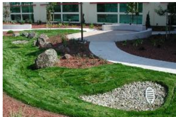
Figure 3-5. Drain rock is used to prevent erosion of this vegetated swale at Zone 7 Water Agency's office building.
