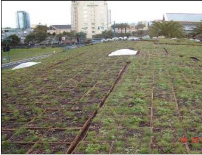
Figure 8-34 Extensive Green Roof in Emeryville
