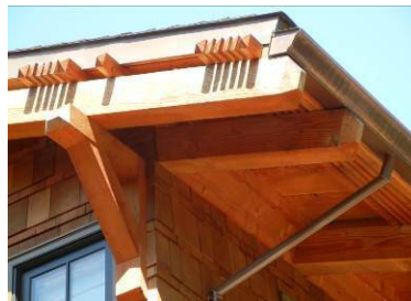
Building with copper flashing, gutter and drainpipe.
