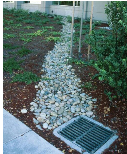
Photo 7-1. Draining roof runoff to a landscaped area is an example of hydrologic source control.
