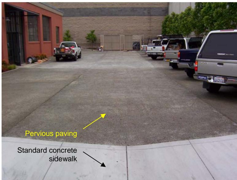
Figure 8-6: Parking Lot with Pervious Pavement, Emeryville
