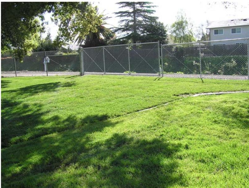
Figure 8-7: Turf block fire access (Source: City of Pleasanton)
