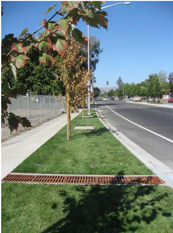
Figure 8-3: Series of non-proprietary tree well filters installed along roadway, City of Fremont
