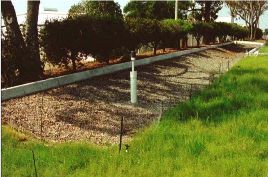
Figure 8-4: Infiltration Trench (Source: California Stormwater Quality Association)
