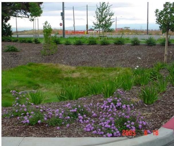
Figure 8-1: Bioretention Area in the City of Fremont
