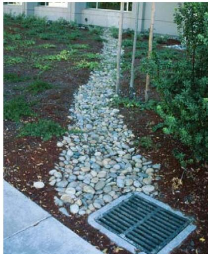
Figure 7-4: Draining roof runoff to a landscaped area is an example of hydrologic source control.
