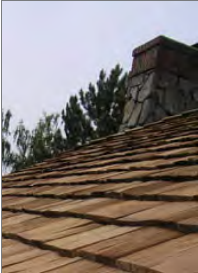
Wood shingle roof Courtesy of Gutter Glove
